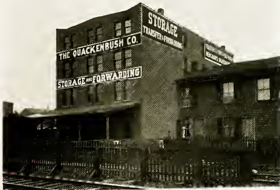
The Quackenbush Co. Storage House Bennett Street
